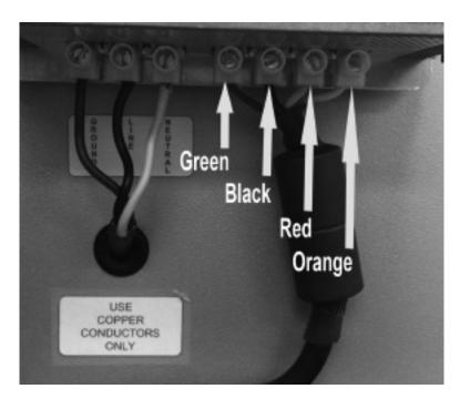
Figure 15 - Cord Reel Wiring Termination
